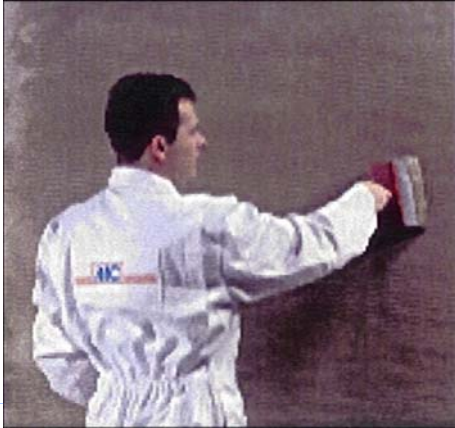
Application of MC-BondAid Plast
