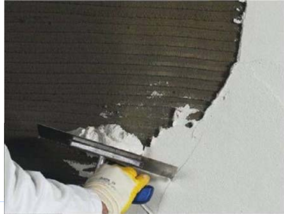
Application of plaster after MC-BondAid Plast
